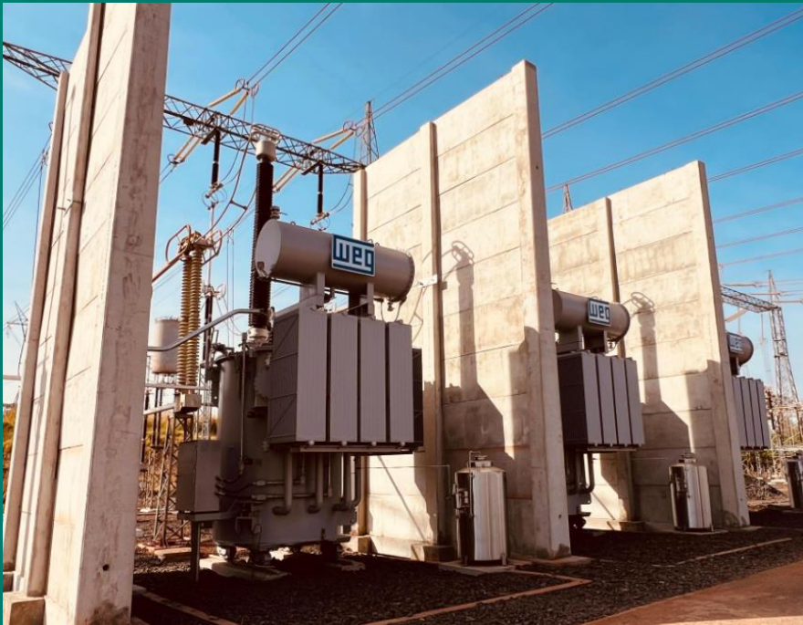
São Simão Substation – new 500kV regulator
