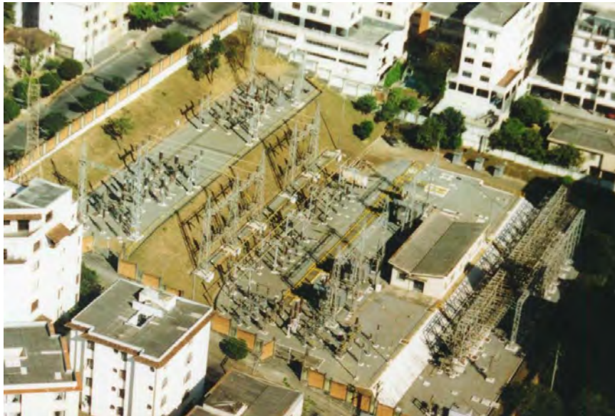
Conventional substation
